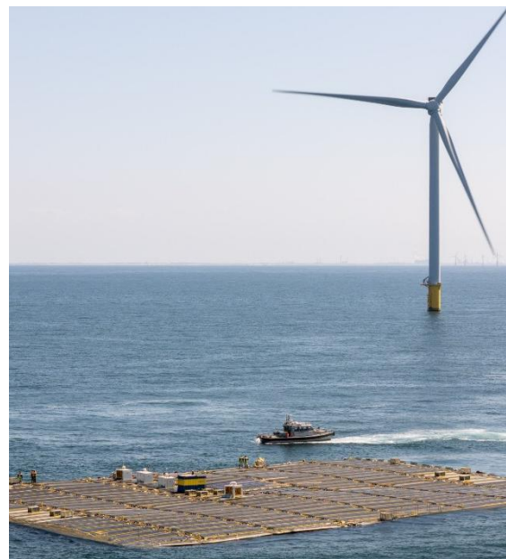
Figure 2 | Offshore solar platform by Oceans of Energy, installed within an offshore wind park in the North Sea.
